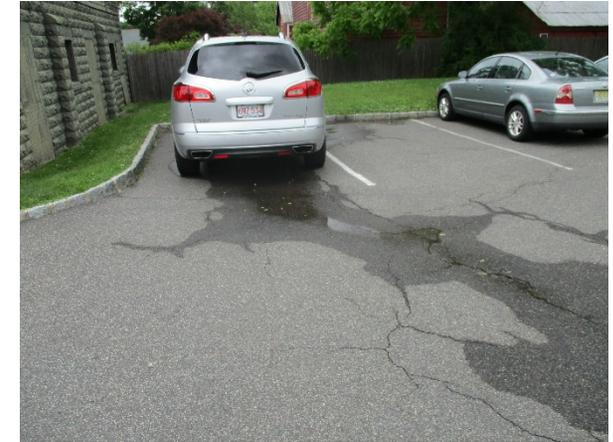
A bioretention system can be installed in the turfgrass area near the brick building to capture, treat, and infiltrate stormwater runoff from the parking lot. The parking spaces east of the entrance can be converted to pervious pavement to help capture additional stormwater runoff. A preliminary soil assessment suggests that more soil testing would be required before determining the soil's suitability for green infrastructure.
