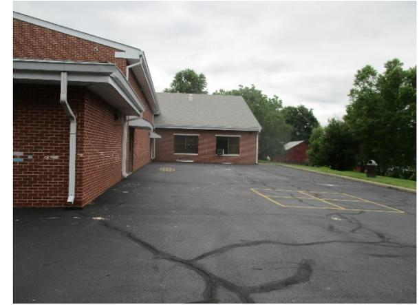
A bioretention system can be installed in the southwest courtyard to capture, treat, and infiltrate stormwater runoff from the building's roof. Planter boxes can be installed on the west side of the building to manage stormwater and beautify the area. A preliminary soil assessment suggests that more soil testing would be required before determining the soil's suitability for green infrastructure.
